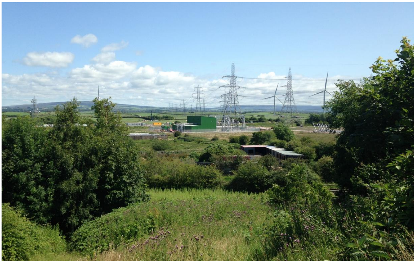
Image 3.5 Existing Middleton 400 kV Substation (Source: National Grid)
