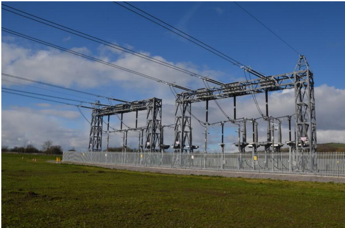
Image 3.9 Existing CSE compound with gantries (Source: ES Chapter 4: Project Description [APP-130](Revision B))
